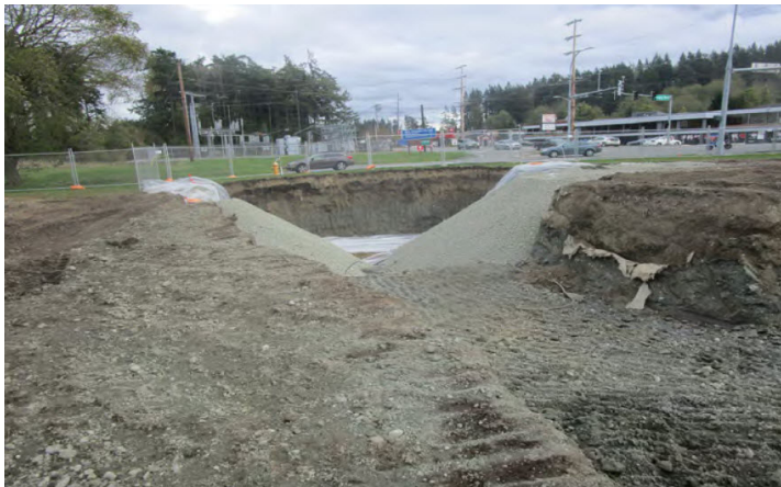
Backfilling (20 OCT 2021)
