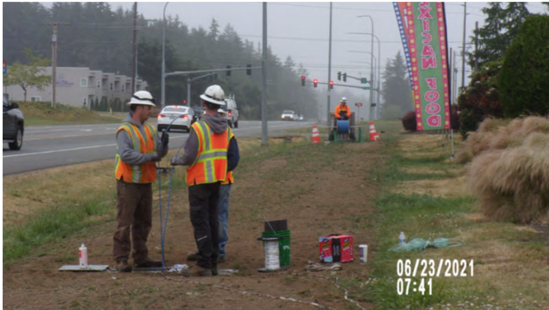
Pulling transducer cables
