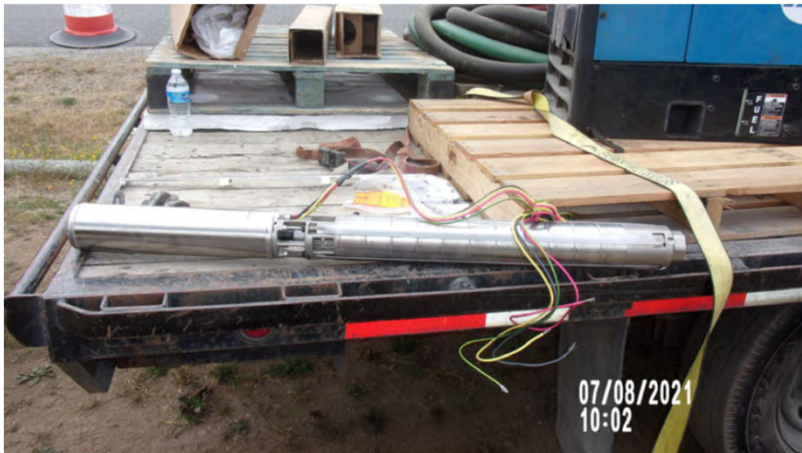
Pump and motor assembly
