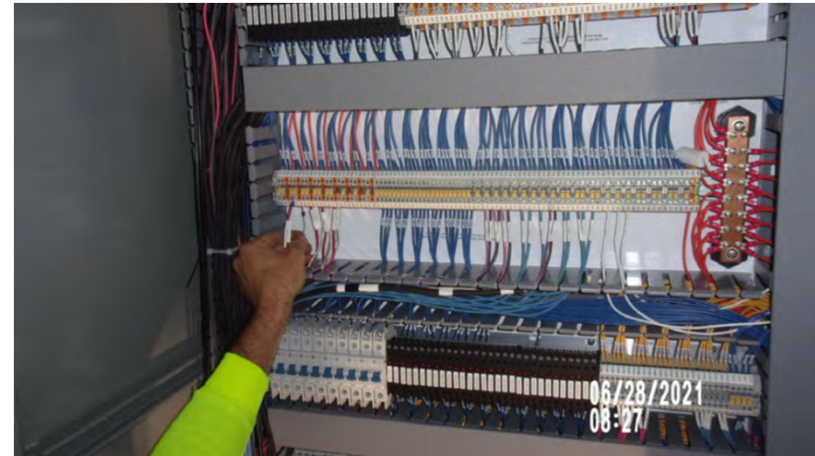
Transducer cables terminating at AOP
